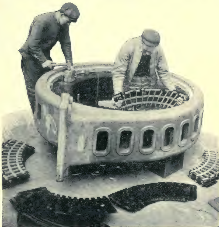
FIG. 91.—Assembling the Core of a Stationary Armature. Mavor & Coulson.
